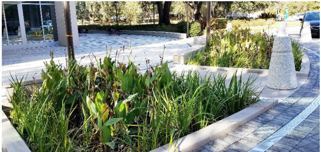
Stormwater planters on south Newell Drive at the Harrell Medical Education Building
