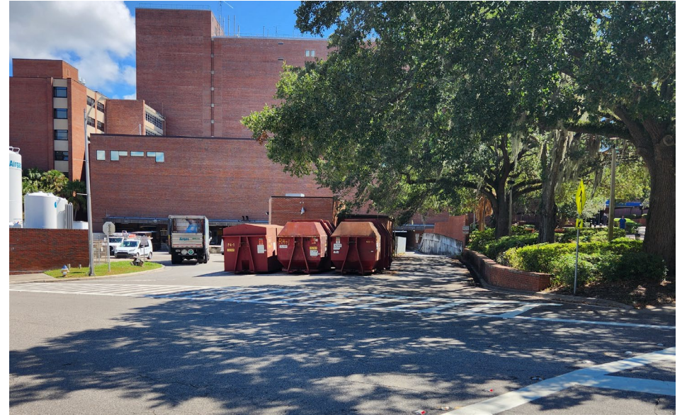
Loading Dock & Tunnel view from Center Drive
