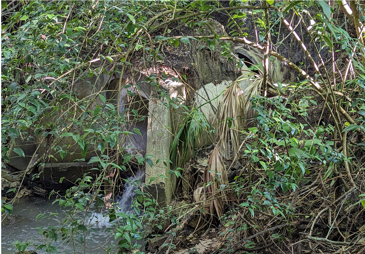
Figure 8. Jennings Creek Headwall Separation
