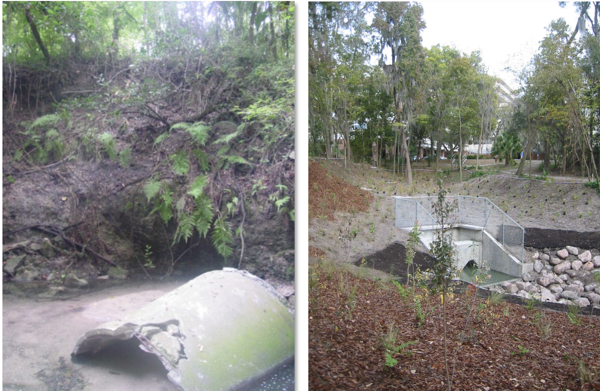
Figure 7. Reitz Ravine Before (2004) and After (2007) Repair and Stabilization
