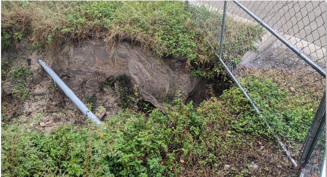
Figure 10. Keys Complex Erosion
