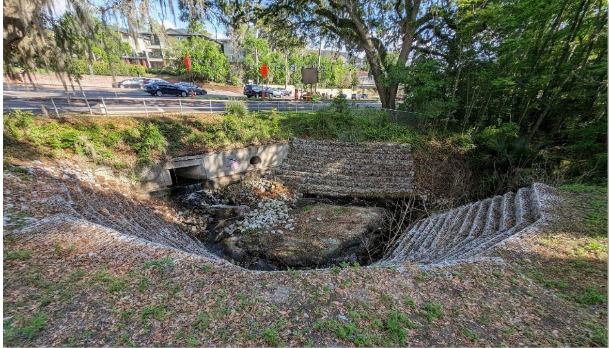
Figure 12. Diamond Creek Bank Stabilization
