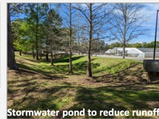
Stormwater pond to reduce runoff
