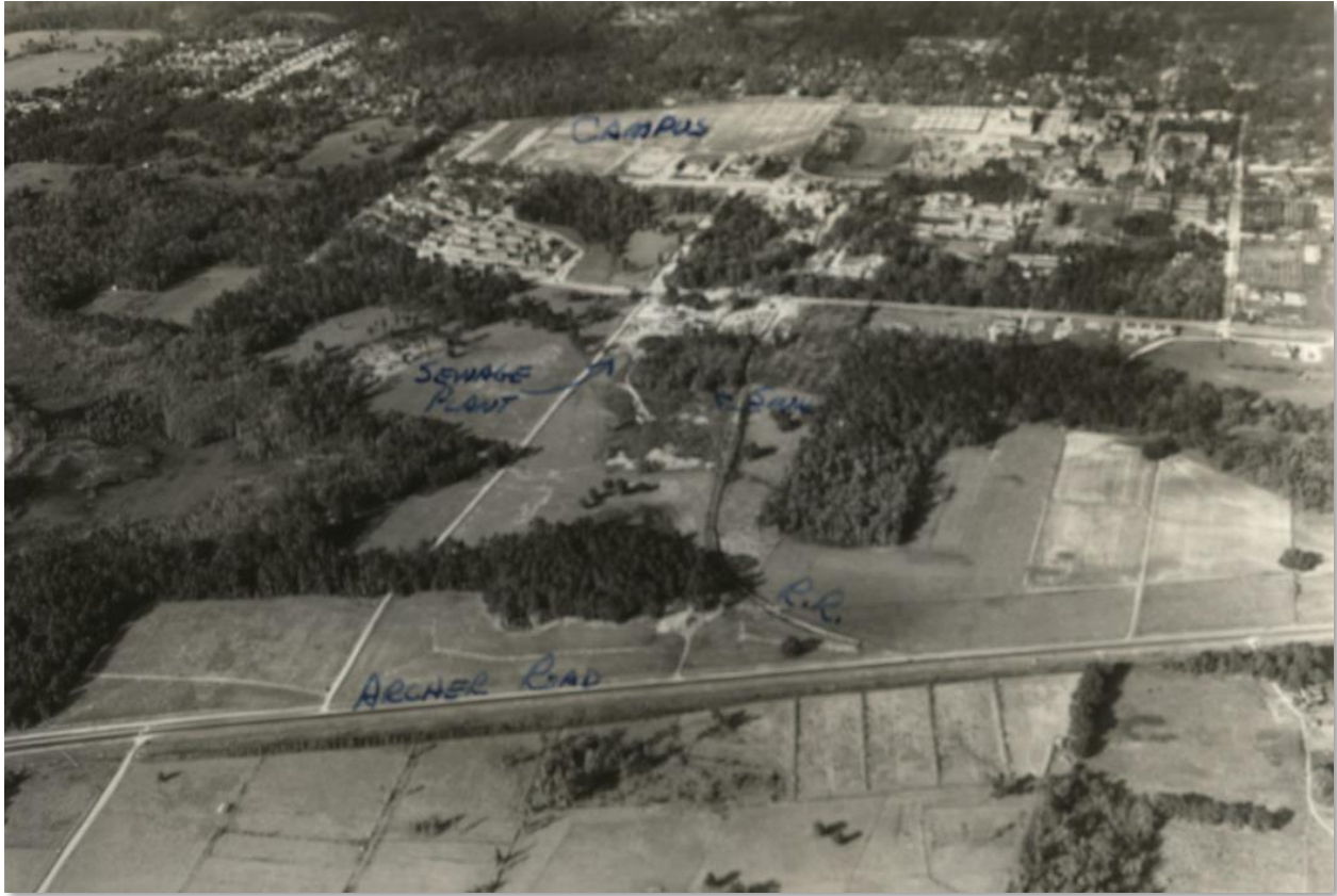
Figure 10. 1947 Aerial Showing Sewage Plant, Railroad Spur, and Sinkhole Drainage Feature
