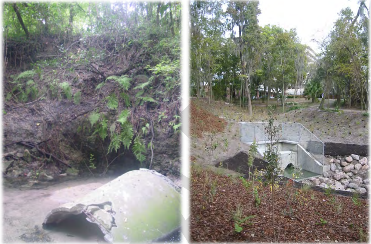
Figure 4. Reitz Ravine Repair and Stabilization Before and After
