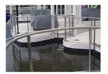
**GUARDRAILS** STAINLESS STEEL WITH METAL MESH INFILL
