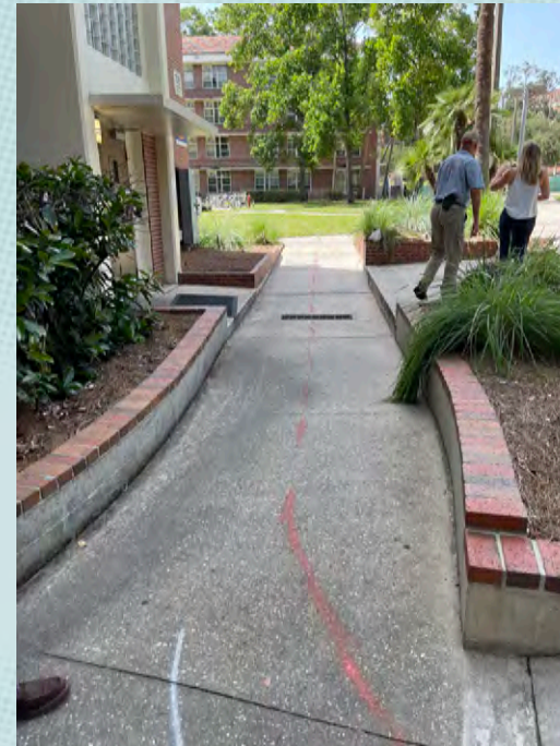
Walk and Drain Inlet at Reid Hall
