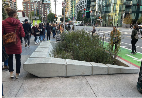
SEAT WALLS CAST IN PLACE CONCRETE
