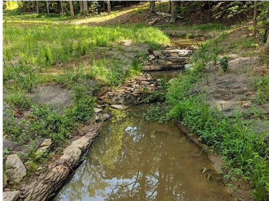
Examples of extreme erosion alleviated with native materials and native riparian plantings
