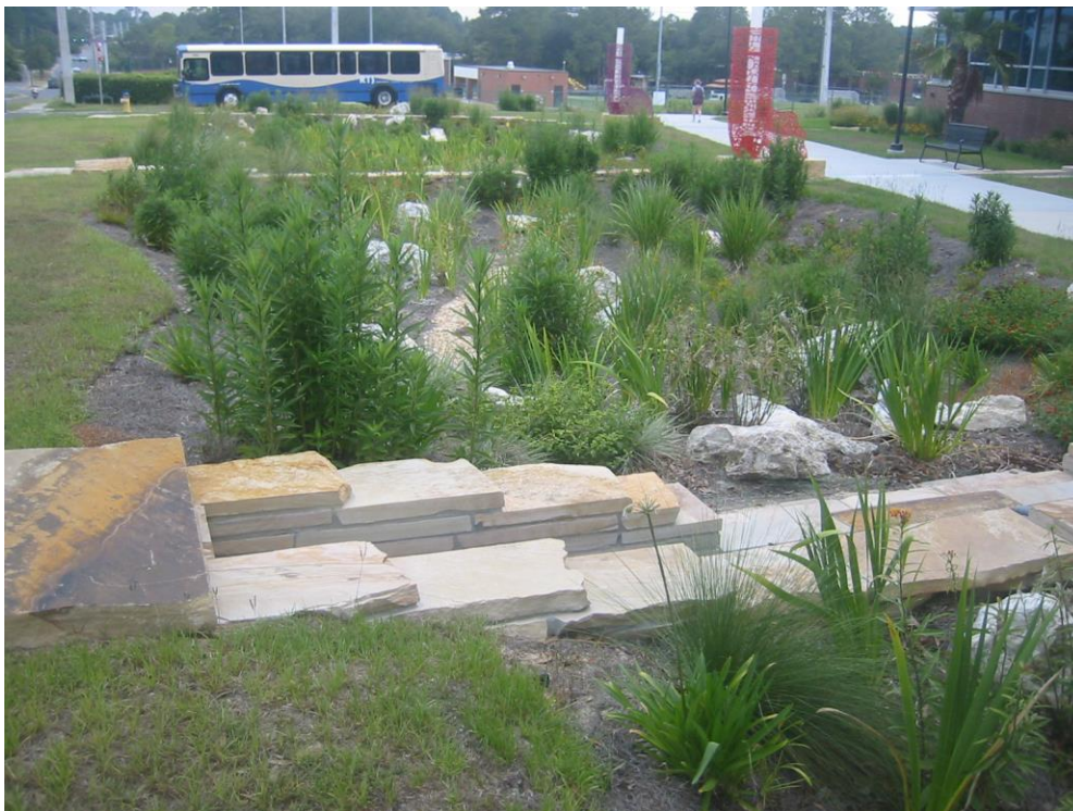
This example illustrates a bio-retention (rain garden) stormwater treatment in front of the Southwest Recreation Center.
