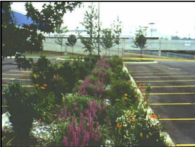
This example illustrates a bio-retention (rain garden) stormwater treatment in a parking lot.
