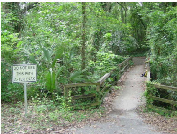
Bridge over Ravine's Creek
